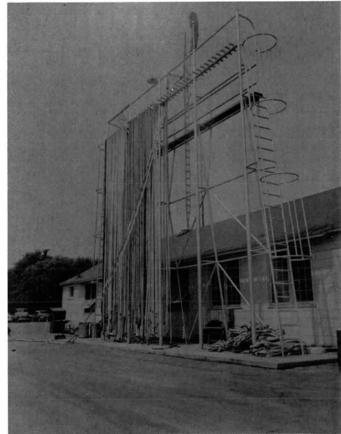
Figure A-5-4(d) Hose drying tower for forestry hose.
