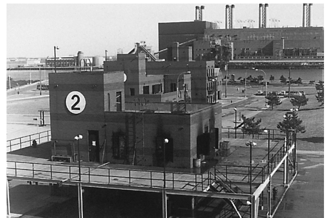
FIGURE 10.1.1 Burn Building with Raised Open-Grid Walkways Level with the Second Floor. (Courtesy of New York Fire Department Fire Academy, New York, NY.)
