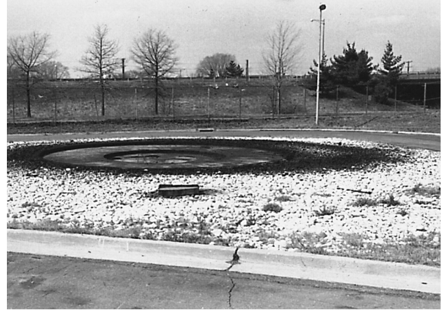
FIGURE 13.2.2 District of Columbia Fire Department Flammable Liquid Pond. Note the Heavy Stone Surrounding Pond. (Courtesy of District of Columbia Fire Department, Washington, DC.)
