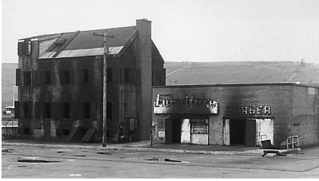
FIGURE 9.9 Both Flat and Sloped Roofs Can Be Designed into a Burn Building. (Courtesy of Nassau County Fire Training Academy, Old Bethpage, NY.)
