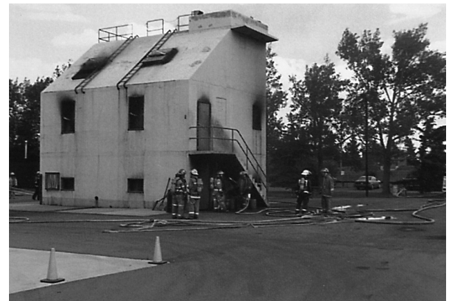
FIGURE 10.1(b) Burn Building with Provisions for Basement Fires and Roof Ventilation. (Courtesy of Alberta Fire School, Edmonton, Alberta, Canada.)
