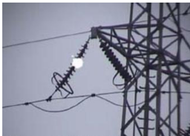
Figure A.28 – Failing external insulation –Example 1
